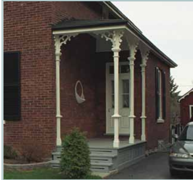
The decorative details on the porch are well handled and appropriately scaled Victorian details.
