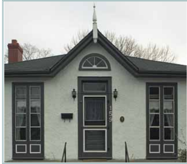
The facade has a centre door with transom above flanked by French windows and front gable with fanlight.
