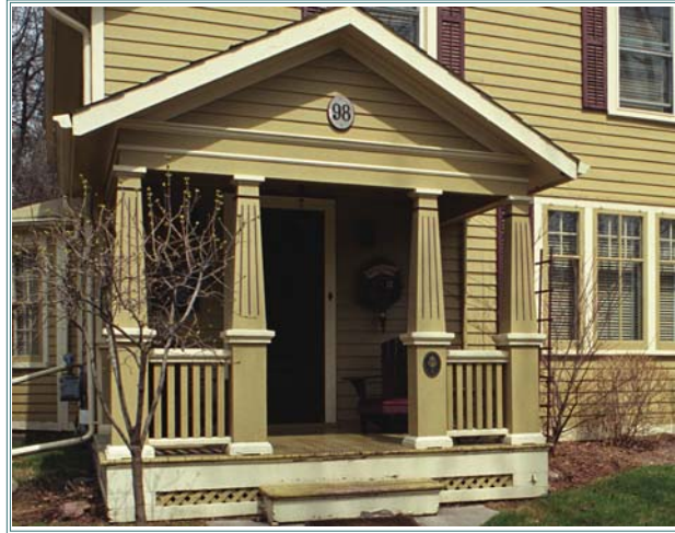
This simple house is adorned by a generous front porch with wood tapered columns. The columns, while simple, have an interesting wood detail replicating flutes.
