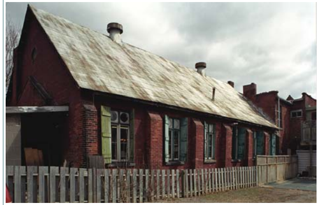
The rear extension of the YMCA measuring thirty by sixty feet was used as the lecture hall.
