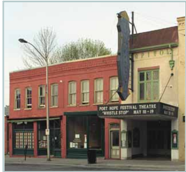
The northern most unit was originally William Stevenson's tailor shop later sold by his son, Charles, to Famous Players in 1930 for construction of the Capitol Theatre.
