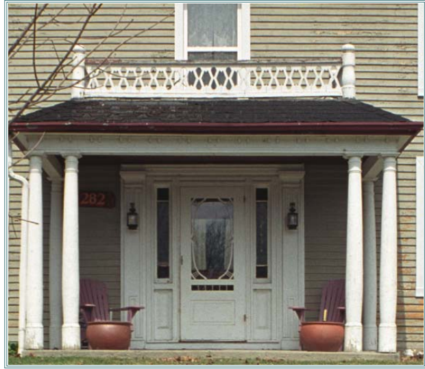
The main door has thin recessed sidelights but no transom panel.
