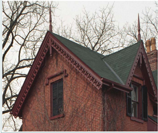
The bargeboard on the gables with pinnacles and drops and the window headers and shutters are noteworthy features of the Billiard House. Emphasis on verticality, multiple gables, decorative bargeboard and finials are typical details of the Gothic Revival style.
