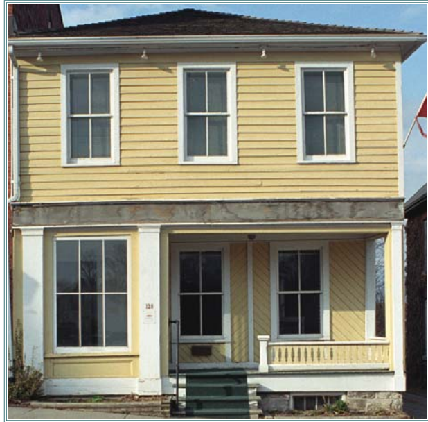
The building recently underwent a facelift. It appears to have evolved from a standard three bay design but at some point the east and centre thirds were recessed. The brackets to eaves may have also been a later addition. At one time a small shop was connected to the east wall of the house visible in a photograph from 1878 in the Clayton Collection. In the Insurance Underwriters Plan of 1901, it was listed as a harness shop. It has since been removed.
