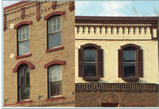
The R.C. Smith Block (48-60 Walton Street) and this building use similar segmental window hood in cast iron and plain cast iron sills. Both buildings incorporate an ornamental brick frieze along the cornice. The modern front brick treatment of the lower front gives the building a less historic character than the two earlier shop fronts seen in archival photos.
