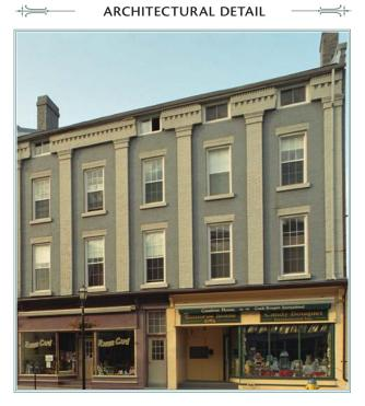
The mid-19th century block with ornamental brickwork to cornice and frieze has been altered by later windows punched through the wall to light the attic storey in the eastern three quarters of the block.
