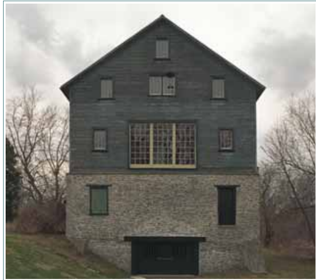
The large multi-paned window was added to the north wall in the 1920's when the Mill House was used as a summer arts school.
